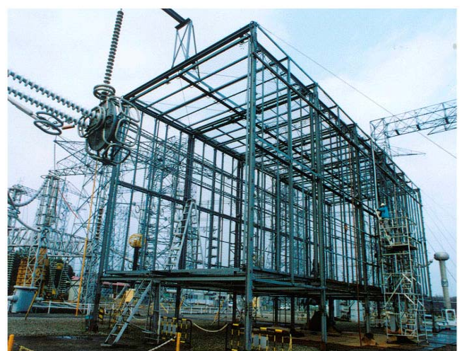
Corona cage at Shiobara Testing Yard
