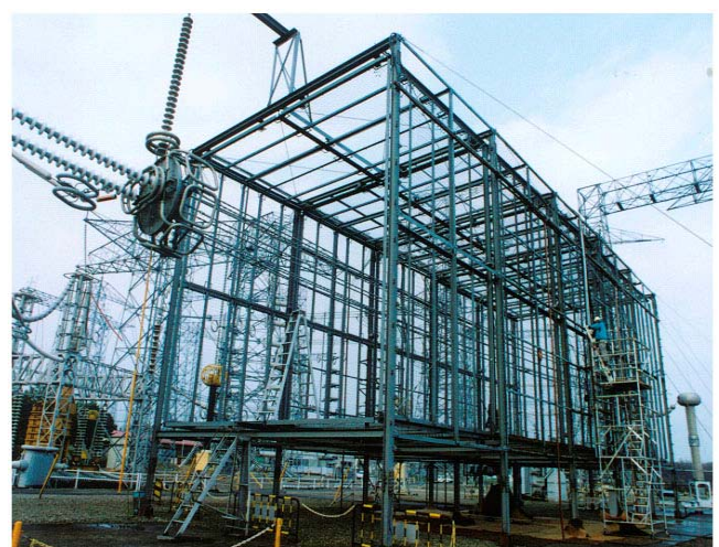
Corona cage at Shiobara Testing Yard
